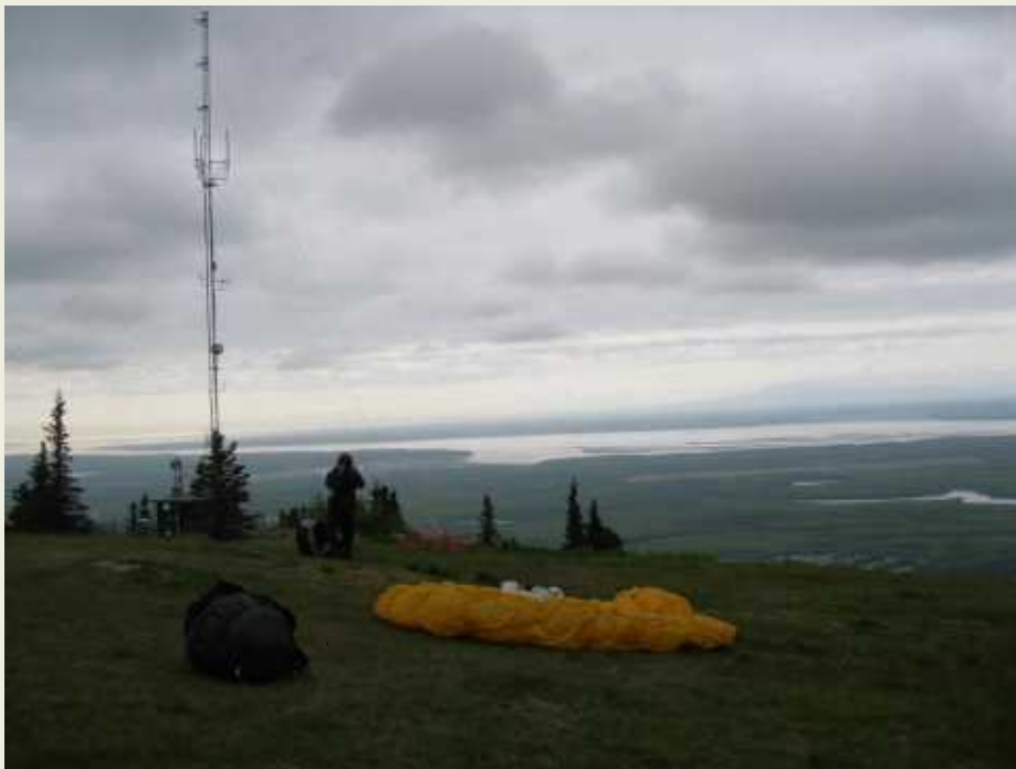
Lower launch, 1900' MSL - next to the radio tower, looking out at Cook Inlet
